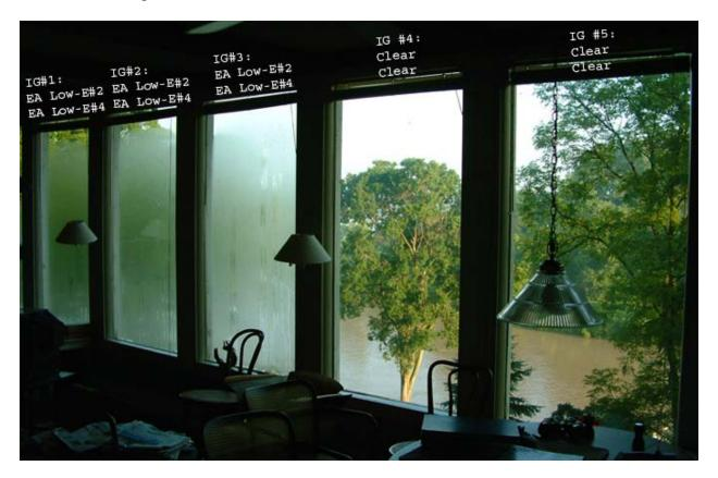
First surface condensation on 3 high performance North elevation, river facing, windows, Ohio, 7:30 a.m in June. Still air, 70 °F, 85% Relative Humidity, 65 °F Dew Point. No air conditioning.
